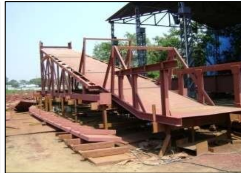
Tripper Structure Platform
