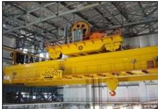
Crane Girder for Capacity 400 and 60 T Span 32M Assembly at HEC
