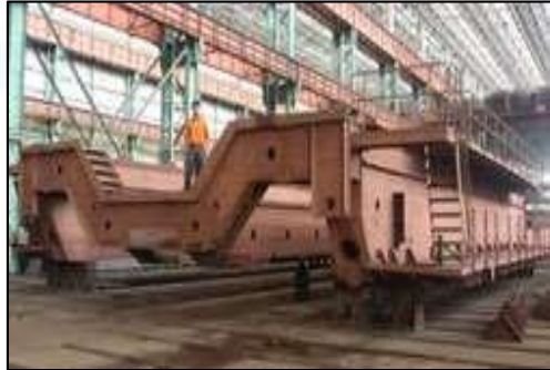
Fabrication of 4 Girder Ladle Crane (180 T capacity)
